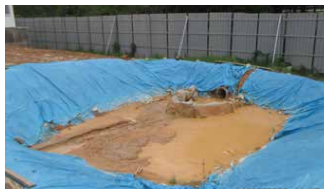
Silt Trap on Construction Site Reducing Water Pollution
